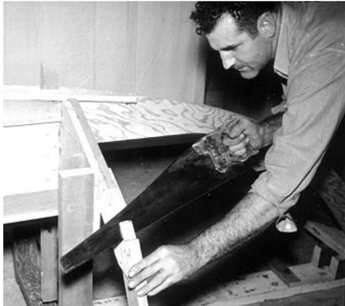
The forward frame is beveled so that the chine will have a flat landing.
