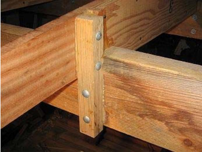
**T**he tip of the stem is referenced from the set-up level, aligned on the centerline and blocked to the base member. Each framework member is then blocked to the form or to one another to prevent movement; all must be aligned and held in place during the entire construction process.
